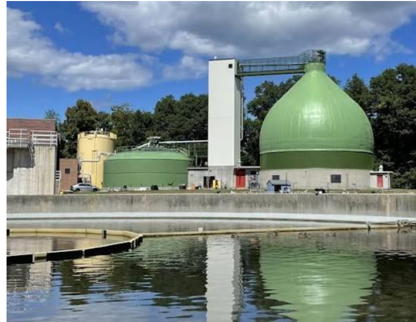
Nashua Wastewater Treatment Facility
