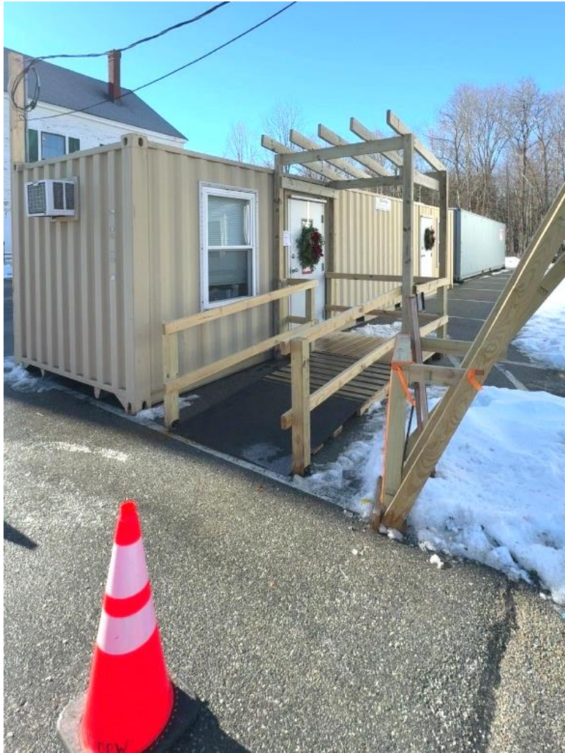
December 2025 – Mont Vernon temporary town hall, two shipping containers placed in the town hall parking lot to relocated staff while hazardous mold is remediated.
