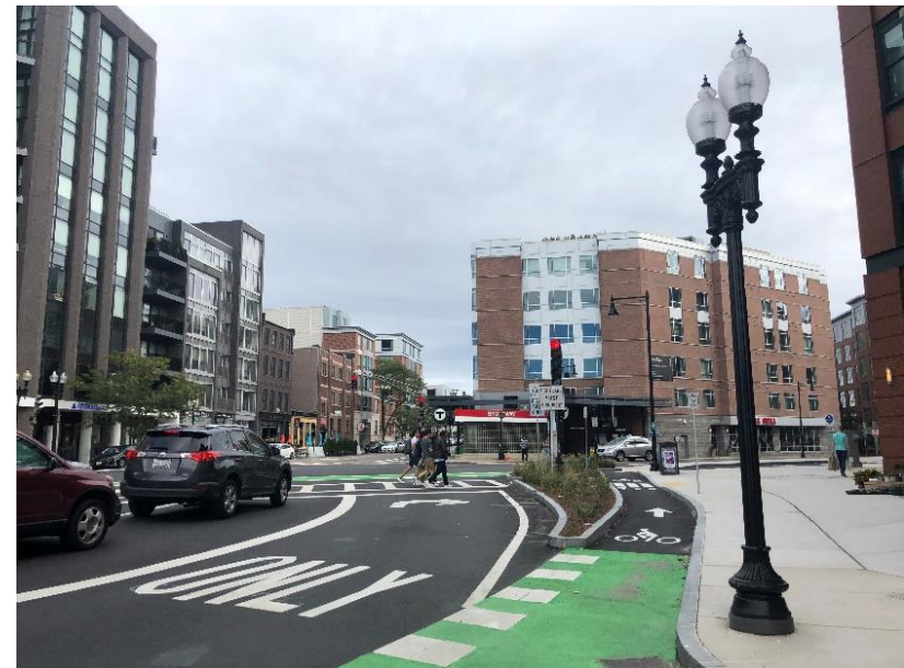
The photo above is a picture of a section of Commonwealth Avenue in South Boston showing a protected bike lane at an intersection separated by a street buffer together with a sidewalk buffer.
