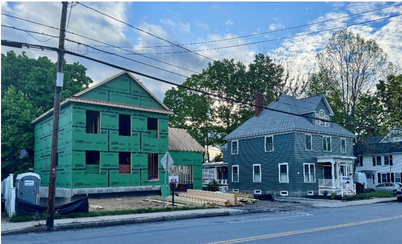
A single family in-fill house under construction in a historic Nashua neighborhood.
