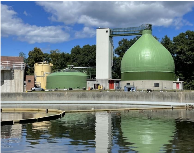
Image of the Nashua Wastewater Treatment Facility
