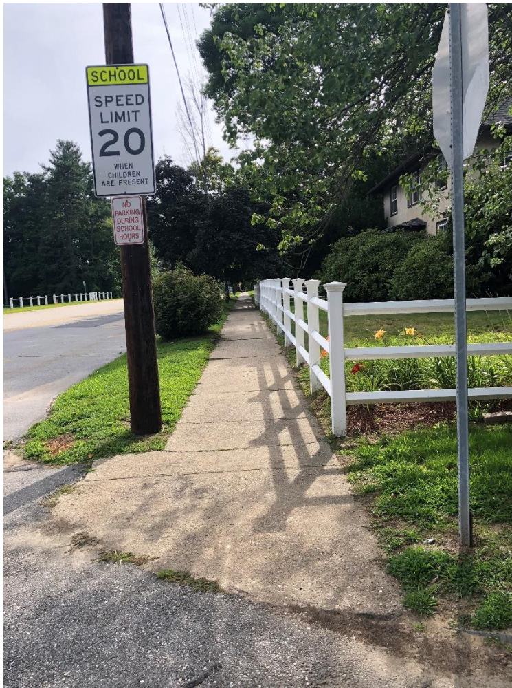
Typical Sidewalk in a Residential Area with grass panel
