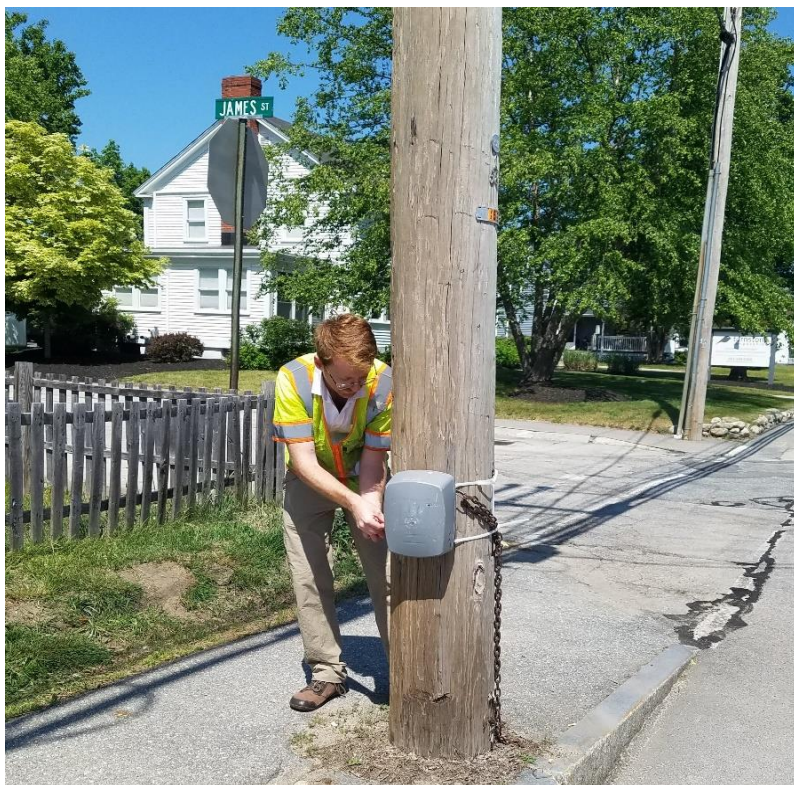
Installing a bike/ped counter in Milford
