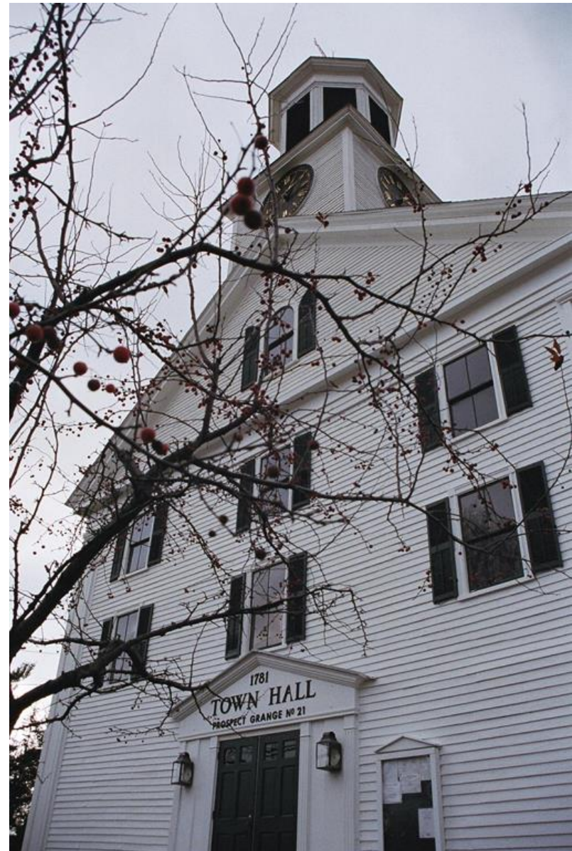
Mont Vernon's Town Hall was closed in 2025 due to toxic mold
